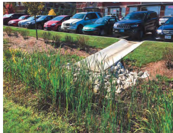
Parking Lot Stormwater
