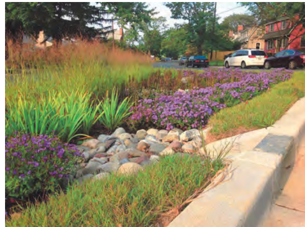
Rain Garden / Bioretention
